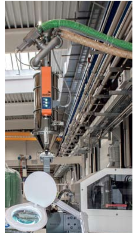
The de-dusting modules enable the use of regrind without loss of quality. The dust is automatically separated into the central filter in a separate room. (Image: motan-colortronic)
